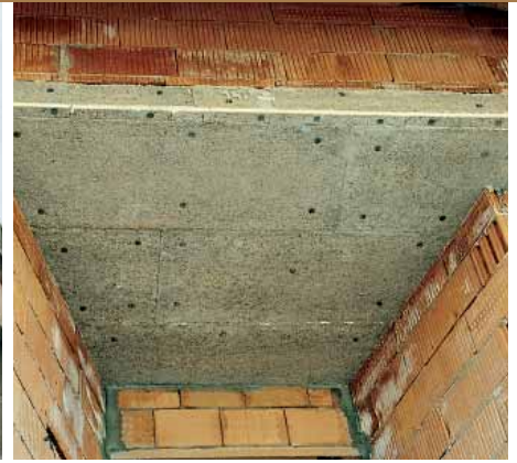
Figure 3 To insulate this thermal bridge, Celenit P3 panels, 35mm thick, were used fixed with plastic anchorages.
