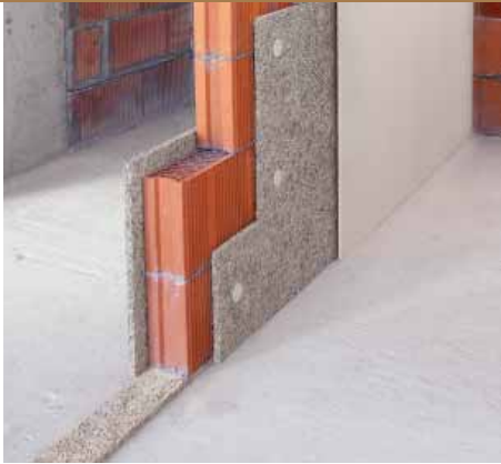
Figure 4 Acoustic insulation of a wall in Poroton® blocks 12 cm thick.
