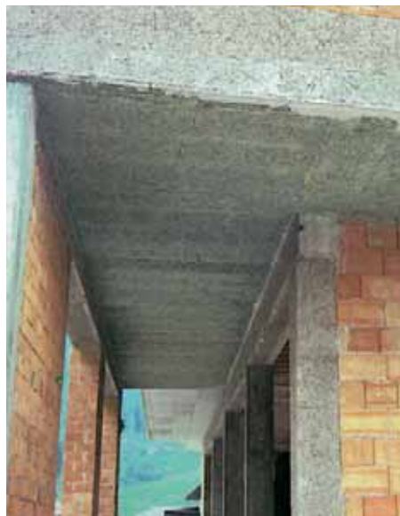
Figure 5 An arcade insulated with Celenit P3 panels, 50 mm thick, placed on the containment formwork before the casting - this operation produces particularly economic results with regard to the reduction in energy consumption and the protection of the structures.
