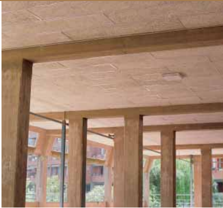
Figure 1 Insulation of arcades in residential buildings using Celenit P2 facing panels mounted on metal profiles in adherence to the flooring.
