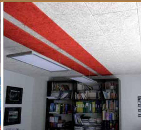
Figure 3 Office - Celenit headquarter - Tombolo (Italy) Celenit AB with two suspended stripes of Celenit ABE, 25 mm thick. Chamfered on all sides.
