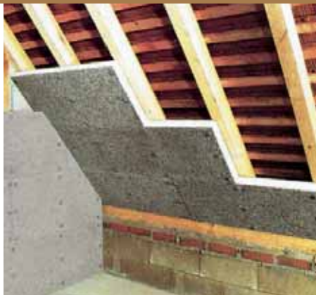
Figure 2 Insulation under beams using Celenit P3 panels.
