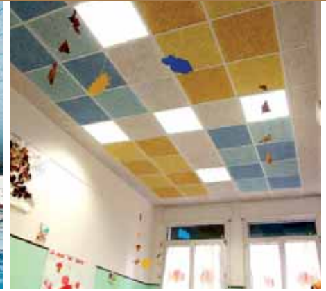
Figure 3 Kindergarten - Cittadella (Italy) Celenit AB, 25 mm thick. For visible T-shaped profiles.
