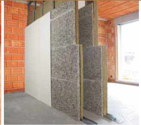
Figure 9 Acoustic insulation of double metallic structure with Celenit N panels and plasterboard.
