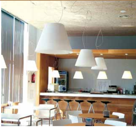
Figure 1 Restaurant - Barcelona (Spain) Celenit AB, 25 mm thick, without painting. Chamfered edges, omega-shaped metal profiles.
