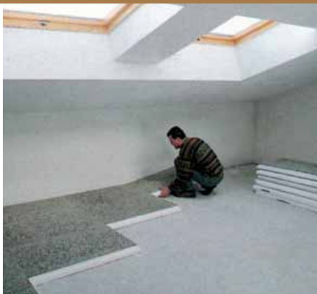
Figure 1 Attic floor insulation using leaf-edged Celenit P2 panels.
