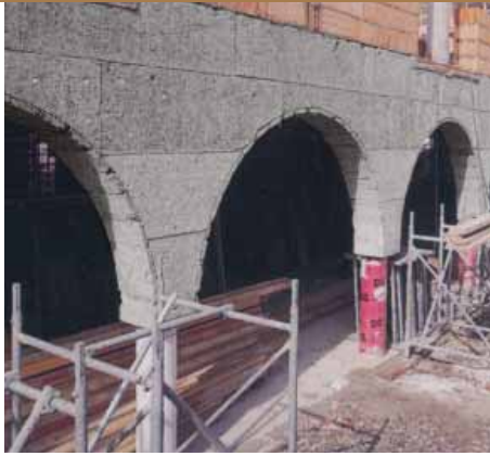
Figure 1 Thermal bridges insulated with Celenit N panels, 35 mm thick.
