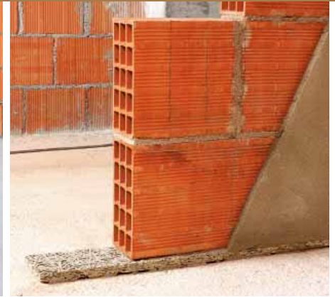
Figure 6 Partition wall insulated with a strip of Celenit N panels. A simple but effective way of interrupting noise transmission to lower floors and adjacent rooms.
