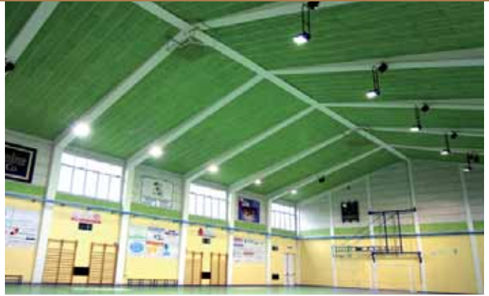
Figure 2 Gymnasium - Breganze (Italy) Celenit AB, 25 mm thick. Chamfered edges, omega-shaped metal profiles.
