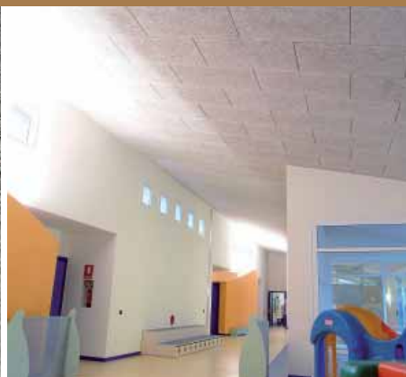
Figure 2 Kindergarten - Valencia (Spain) Celenit AB, 25 mm thick. Chamfered on all sides. Adhering false ceilings.
