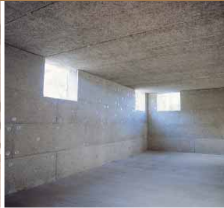
Figure 2 Cellar of a one-family house: the first flooring is a predalle, insulated with 35mm Celenit N panels: acoustic and thermal insulation, some amount of finishing required. The wall was subsequently insulated with 35 mm Celenit P3 panels applied with screw anchors.
