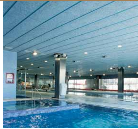
Figure 2 Swimming pool - Girona (Spain) Celenit AB, 25 mm thick. Chamfered edges, omega-shaped metal profiles.
