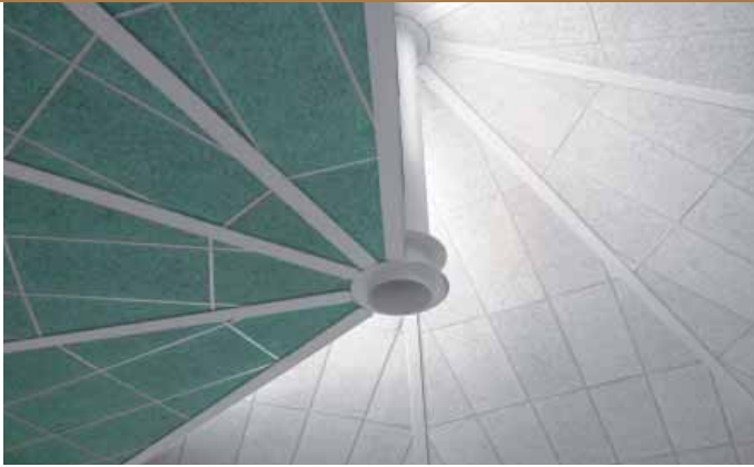
Figure 1 Entrance of primary school – Mestrino (Italy) Celenit AB, 25 mm thick, painted in various colours. For visible T-shaped profiles.
