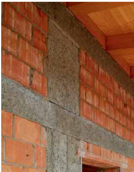
Figure 4 Thermal bridges on inter-floor beams and pillars can be adjusted, at the casting stage, by inserting Celenit N or Celenit P3, Celenit E3 or Celenit G3 panels in the formwork. For this specific use, made-to-measure strips are supplied by the company.
